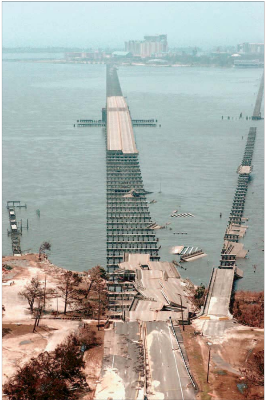
Wrecked bridges, Ocean Springs, MS Sun Herald news photo, Biloxi/Gulfport, MS
