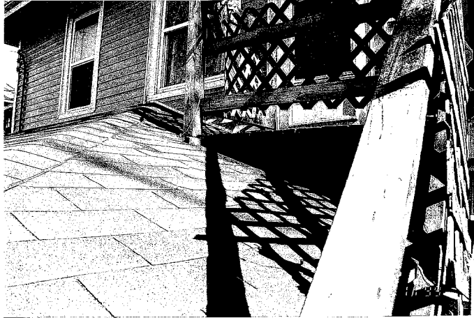
Deck nailed through the roof.
