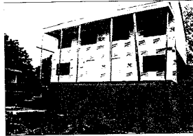
Exterior work at 1470 Constance Street Scattered Site.
