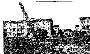
Demolition activity at Florida.
