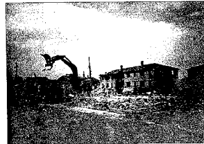
Demolition activity of buildings at Desire Housing Development.
