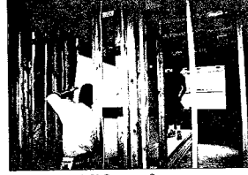
Interior work at 1470 Constance Street.
