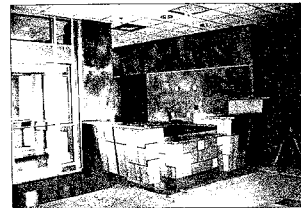
Main lobby and security desk of renovated High Rise.
