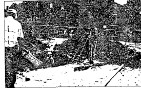
Sewer and water line work done in the Iberville Housing Development.
