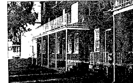
Lead paint abatement in Iberville.
