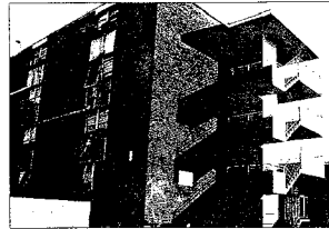
View of existing buildings at Guste Homes Low-Rise.
