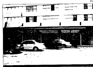
Main entrance to renovated Guste Homes High Rise building.
