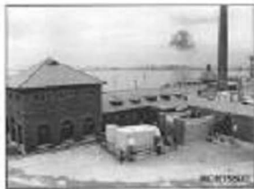
Resource Recovery Waste Water Treatment Facility Deer Island, Boston, Massachusetts
