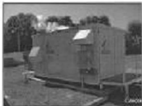
Resource Recovery Waste Water Treatment Facility Portland, Oregon
