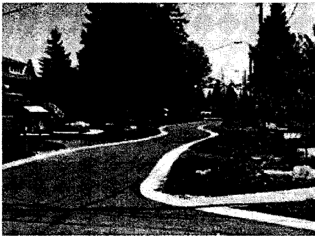
Seattle Public Utilities SEA Streets Site after improvements and drainage retrofit using LID techniques.
