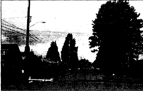
Seattle Public Utilities SEA Streets Site before street improvements and drainage retrofit using LID techniques.
