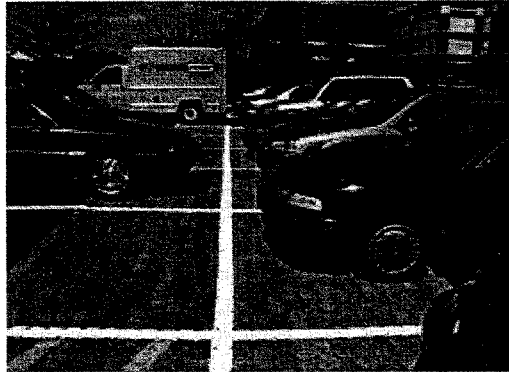
Low Impact Development Center Permeable pavers used in areas of low traffic flow or between parking rows allow runoff water to be infiltrated into the ground without reducing the amount of parking.
