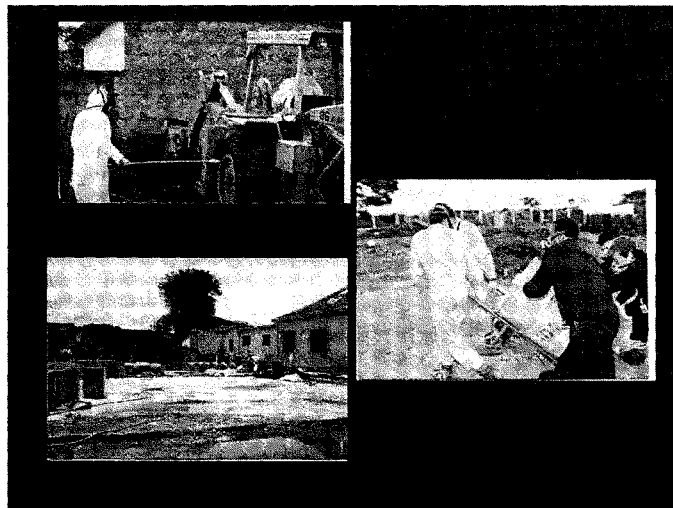
Photos of the scrap yard, demolition of a building and carting of contaminated soil.
