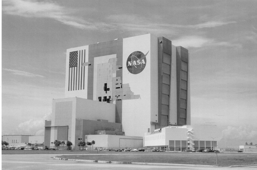
VAB—The massive Vehicle Assembly Building (VAB) at NASA Kennedy Space Center lost about 820 panels during Hurricane Frances. None of the equipment inside the building, was seriously damaged. The VAB is 525 feet tall and is covered by nearly 1,100,000 square feet of insulated aluminum panels and 70,000 square feet of plastic panels.
