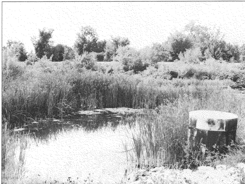
Stormwater runoff from the auto-related businesses on U.S. Route 7 is diverted into a four-acre system of settling ponds and constructed wetlands prior to discharge into Bartlett Brook and Lake Champlain.
