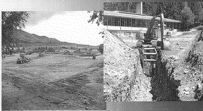
Constructing to grade pad for new hospital and installing utilities onsite.
