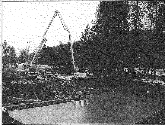
Blackwell Boat Launch concrete placement.
