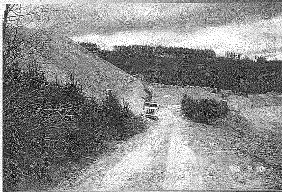
U.S.F.S. Road Relocation and Construction of French Drain
