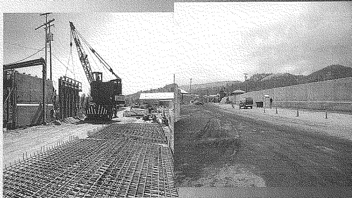
Construction of floodwall with crane and completed floodwall.
