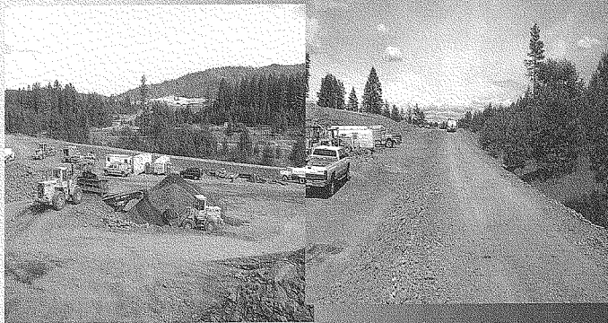
Screening materials to spec. and constructing 10' wide path to grade.
