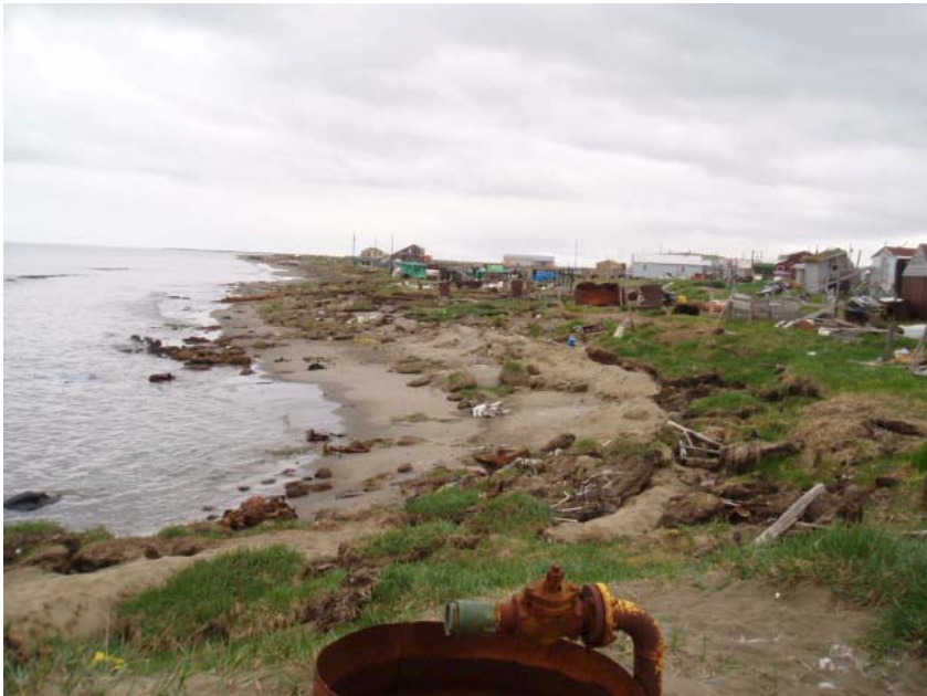
Center of town looking east
