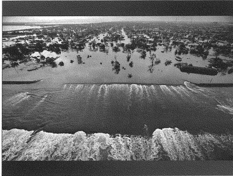
Picture1: Breached levee.
