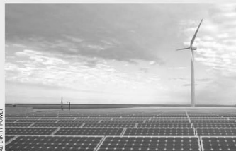
The Atlantic County Utilities Authority dedicated the Jersey-Atlantic Wind Farm, supported by solar power, in Atlantic City, N.J., in December.
