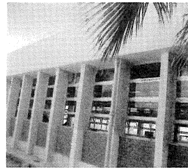
Completed Repair Work At Al Basrah University
