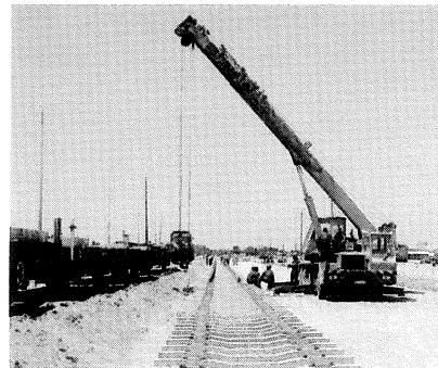
Laying New Track
