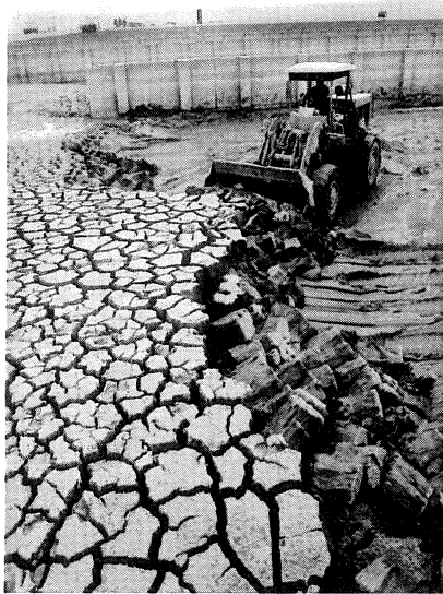
Sweet Water Canal Before
