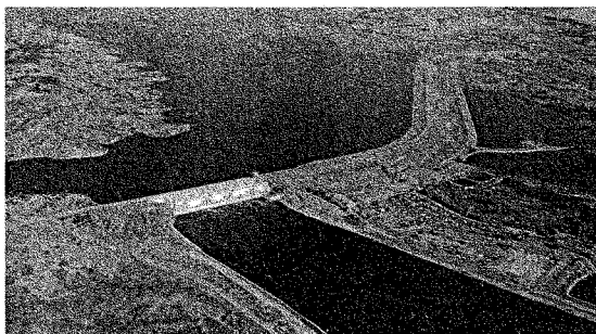
Figure 2: The Big Bend Dam and Lake Sharpe (July 1998)
