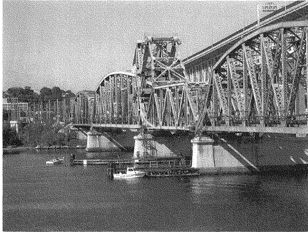
Bridge built in 1919, but increasingly unreliable
