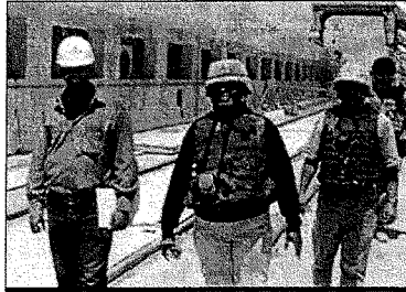
U.S. and Iraqi engineers working together at the An Nasiriyah drainage pump station project. U.S. Army photo by James Bullinger.
