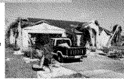
After Hurricane Charley - Home across the street built to older code
