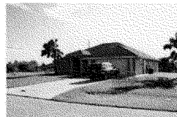
After Hurricane Charley - Home built to newer Florida code
