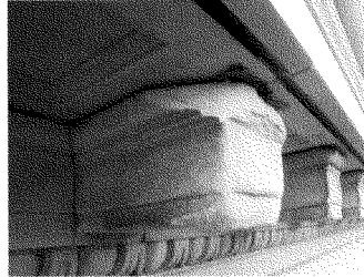
Deteriorated Modillion
