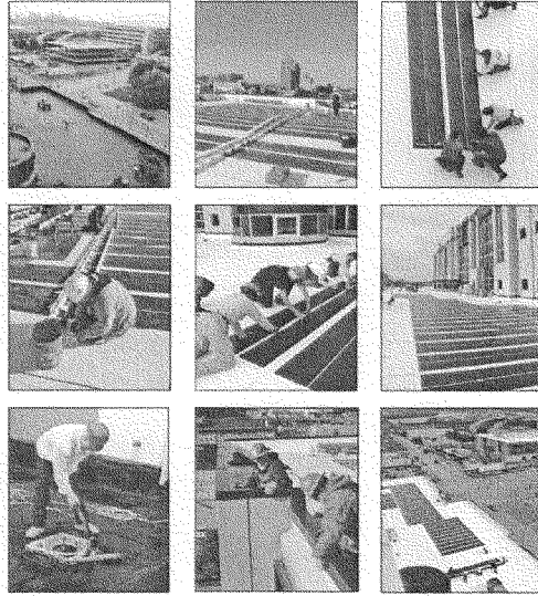
Construction Photos: Robert J. Dole U.S. Courthouse Kansas City, Kansas
