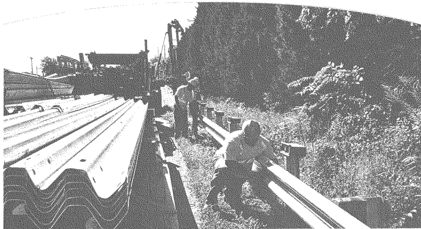
Installing guardrails to improve safety was a goal of several recovery projects.
