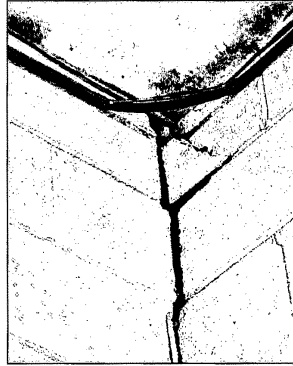
There are many severe cracks inside the academic buildings, which could cause wiring to short-circuit.
