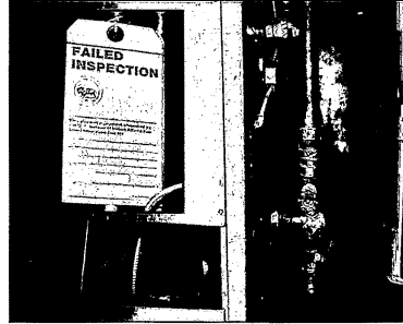
A failed inspection tag, dated 2002, hangs from the continuously leaking boiler.
