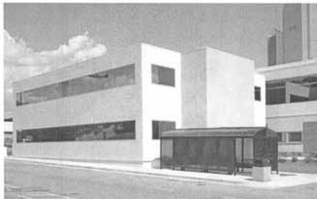
Project by Ramtech
