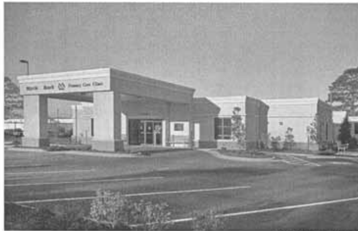
Project by Ramtech
