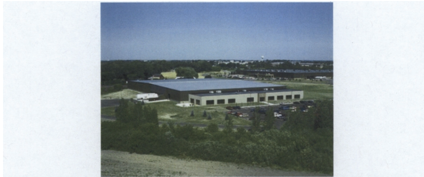
Johnson Controls Li-ion Cell Manufacturing and Battery System Assembly Plant, Holland, Michigan
