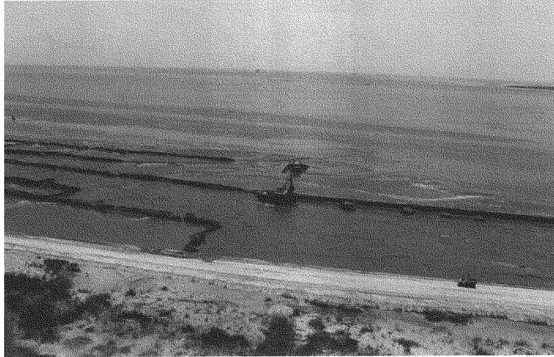
Marsh Buggy Excavator
