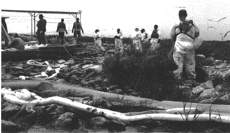
Crews Cleaning Up Oil @ Cat Island
