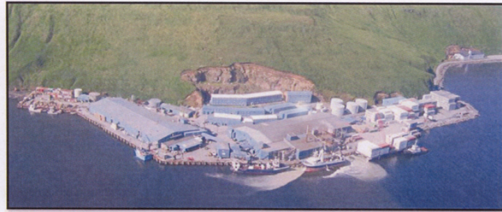
Figure 1. Trident's Akutan Plant in 2012
