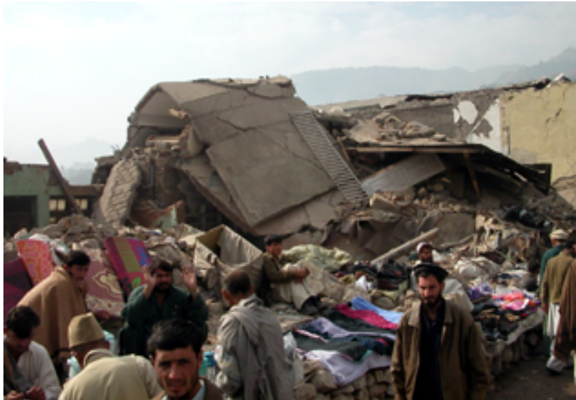
Earthquake destruction in downtown Muzaffarabad
