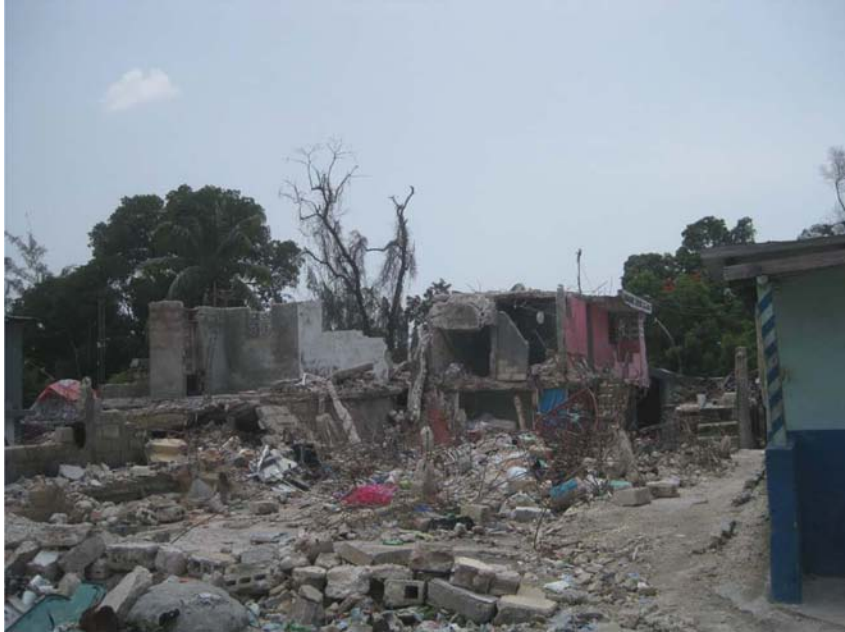
Fig. 9: Even five months after the earthquake, rubble blocks and slows travel on roads in many parts of Port-au-Prince, leading to horrific traffic congestion and continuing to make sections of the city impassable. Rubble removal is the first critical step towards reconstruction; it is a precursor to accessible roads, ports, airports, as well as improved infrastructure such as water, sewage and electrical systems. Until the rubble is removed, Haitians will not be able to return to their pre-earthquake communities. June 8, 2010
