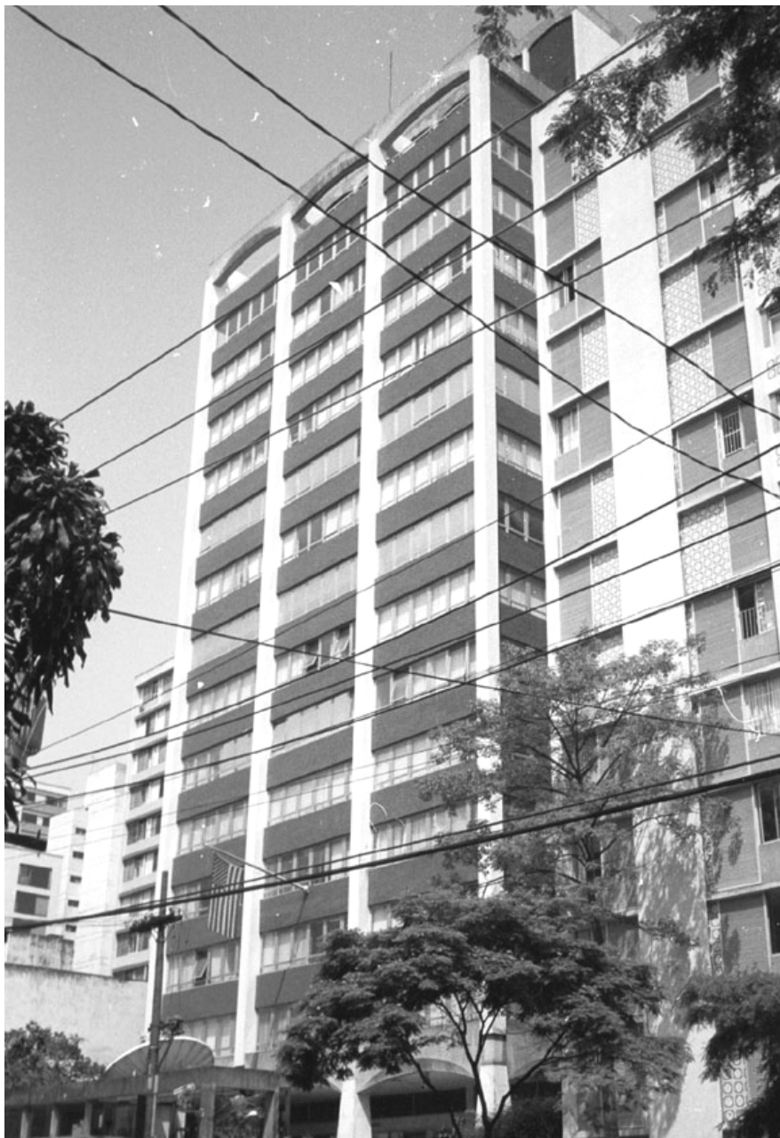
Figure 16: Existing Consulate in São Paulo, Brazil
