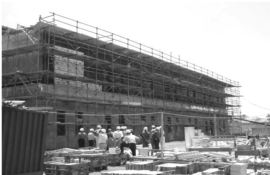
Figure 1: Construction Underway at Site in Kampala, Uganda, as of September 2000
