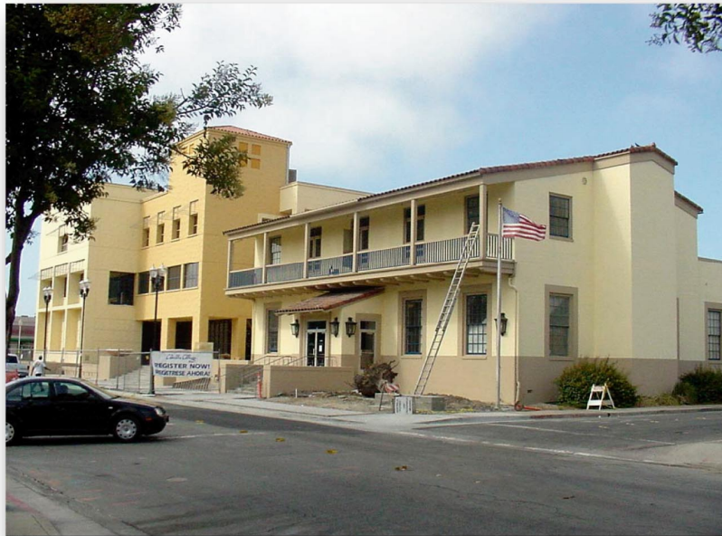
Construction is finishing on the new Cabrillo College campus in downtown Watsonville.
