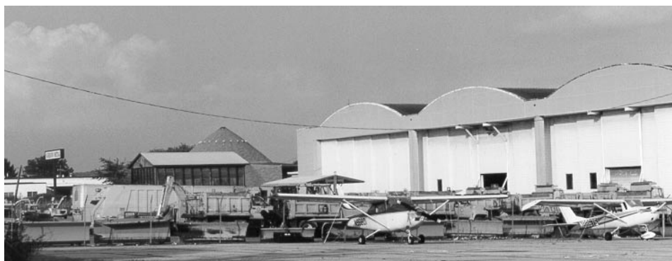
Figure 11: Vehicle Maintenance Facility at Queen City Municipal Airport, Allentown, Pennsylvania
