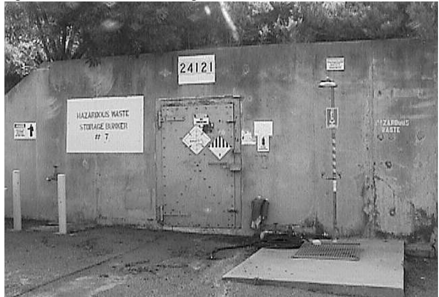
Figure 1: Hazardous Waste Storage Bunker
