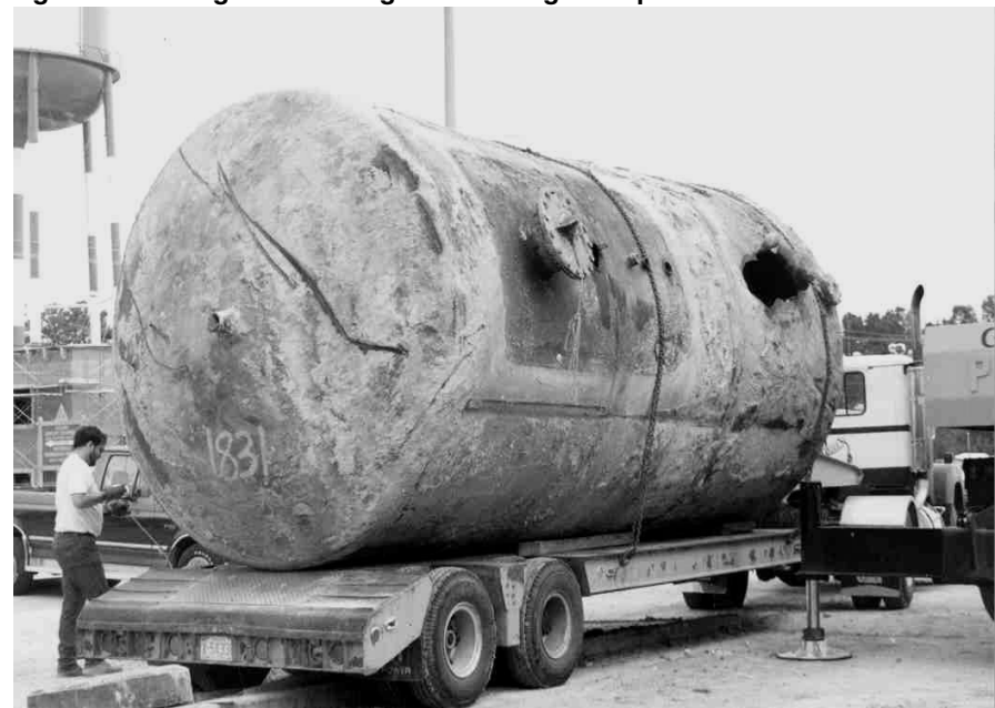
Figure 2: Underground Storage Tank Being Transported After Removal
