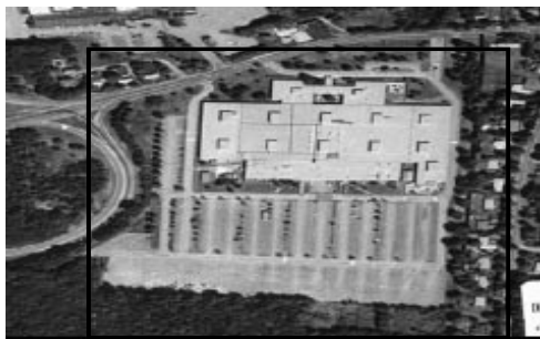
Figure 24: IRS Service Center, Andover, Massachusetts
