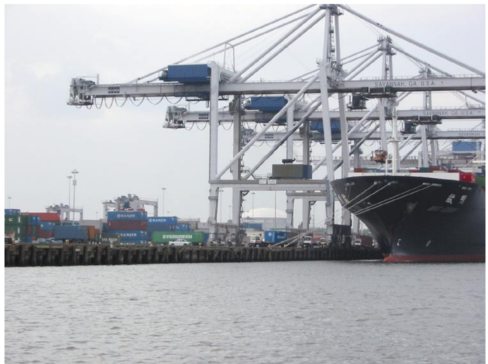
Figure 2: A Commercial Container Vessel and Related Infrastructure at a Seaport
