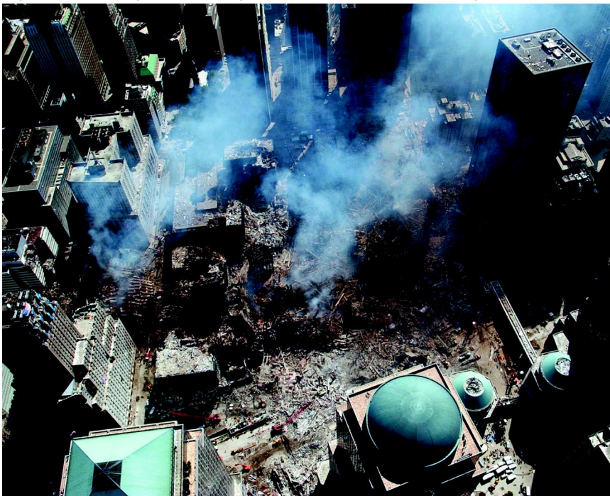
Figure 4: Damage to Buildings from Attacks and Resulting Debris
