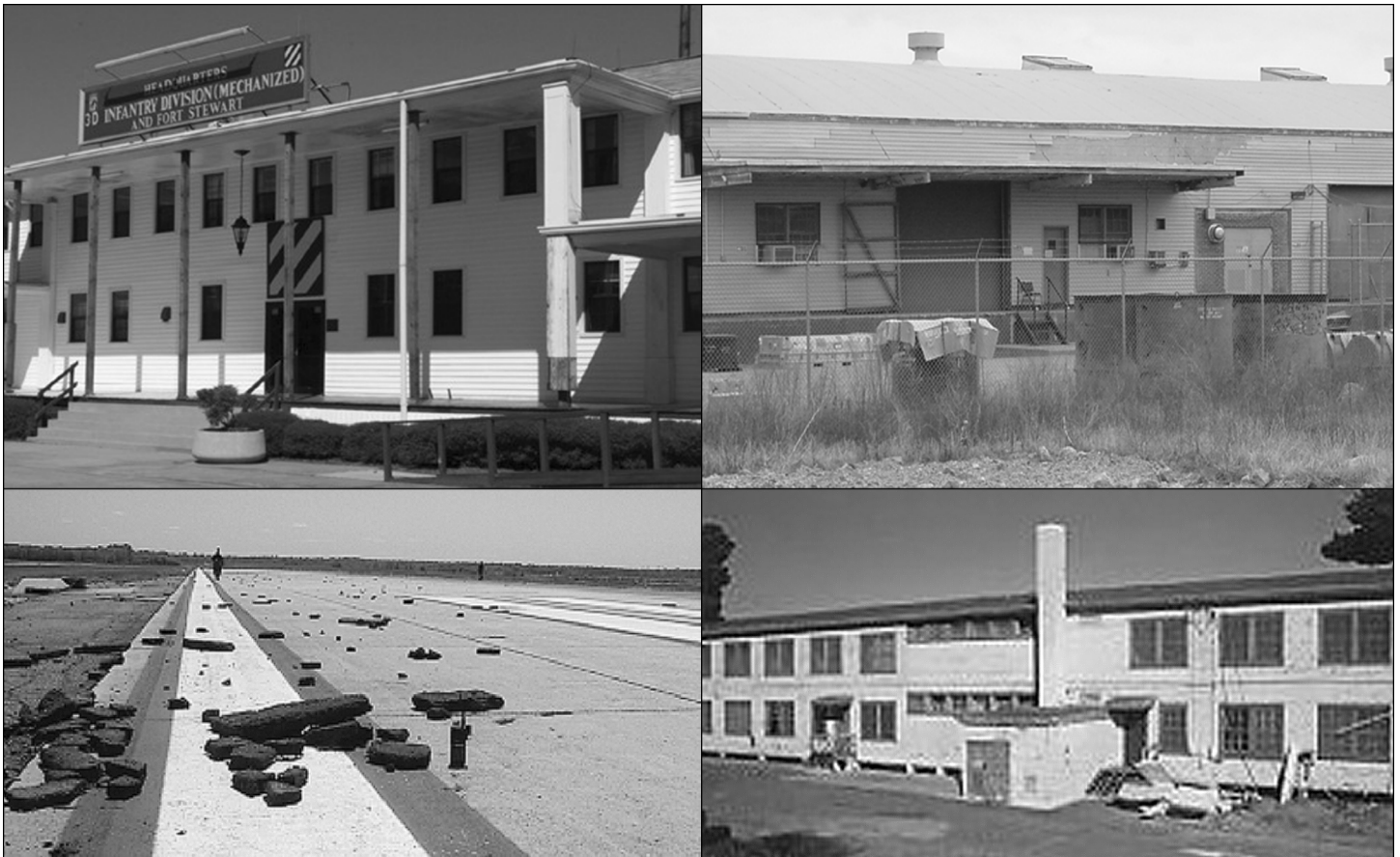
Figure 2: Examples of Undersized or Inadequate Facilities
