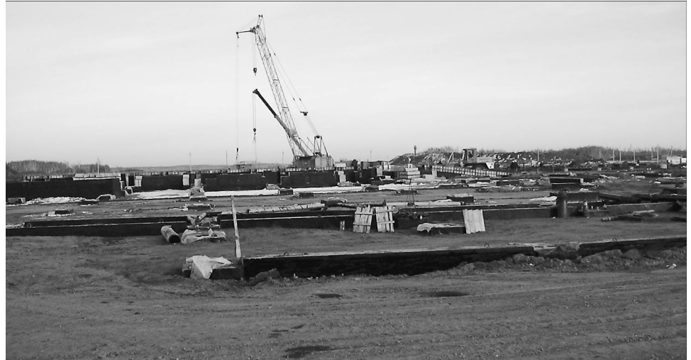
Figure 4: Construction of the U.S. Destruction Building at Shchuch'ye, November 2003
