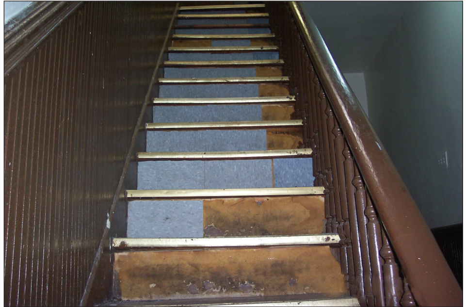
Figure 27: “Newly Tiled” Stairway
