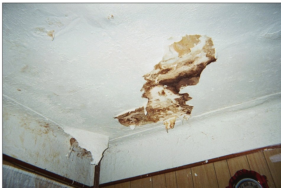
Figure 24: Property 5—"Plastered and Painted" Ceiling
