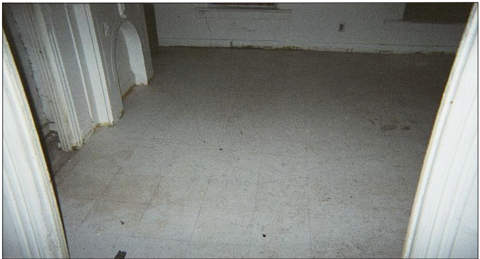
Figure 20: Property 3—"New" Living Room Floor
