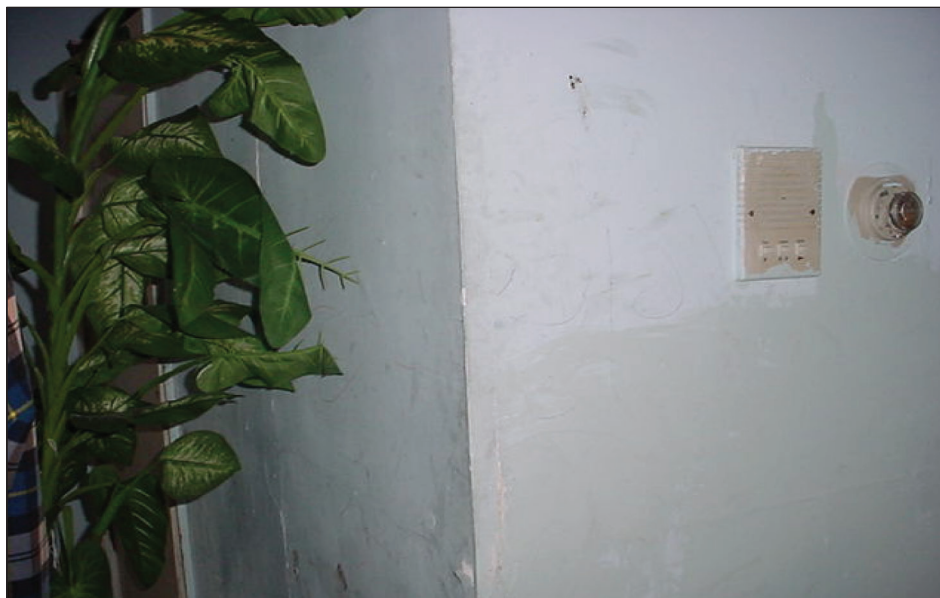
Figure 13: Property 1–“New” Sheetrock® Walls
