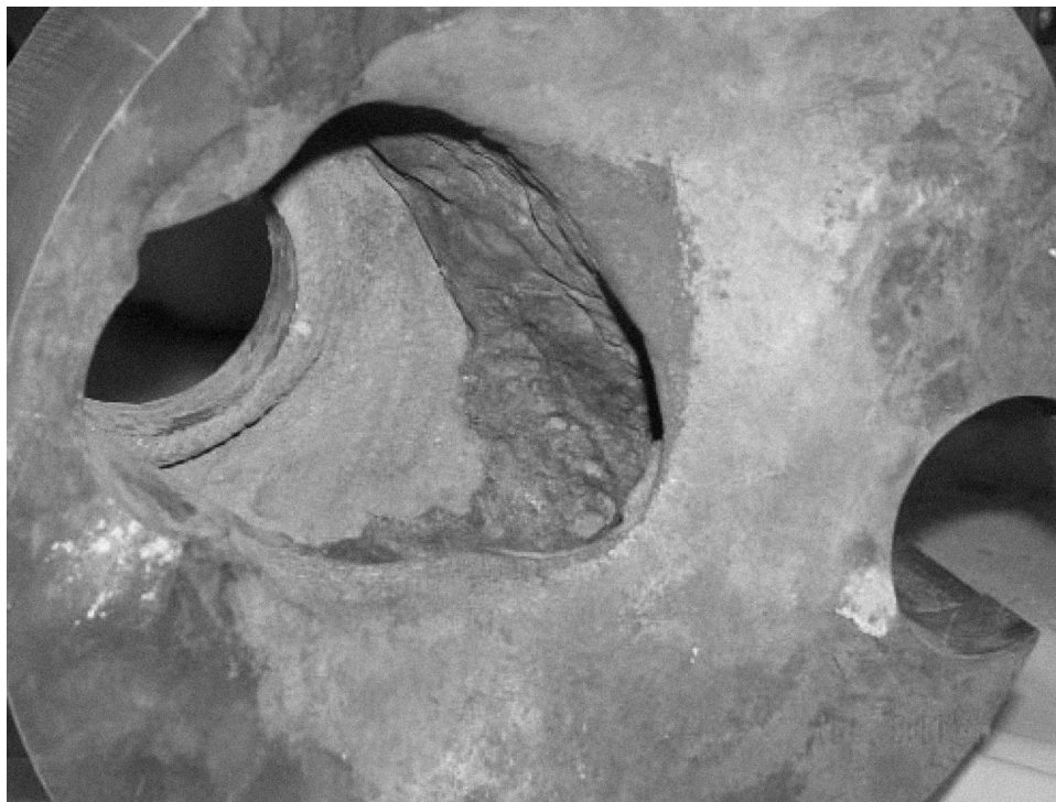
Figure 4: The Cavity in Davis-Besse's Reactor Vessel Head after Discovery
