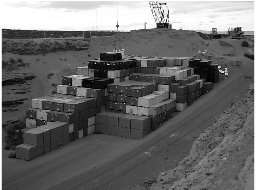
Figure 6: LLRW Disposal Trench at the Richland Disposal Facility
