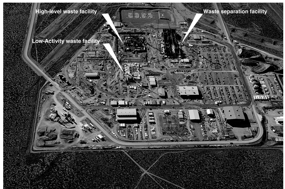
Figure 1: Aerial View of the Waste Treatment Plant, March 2004
