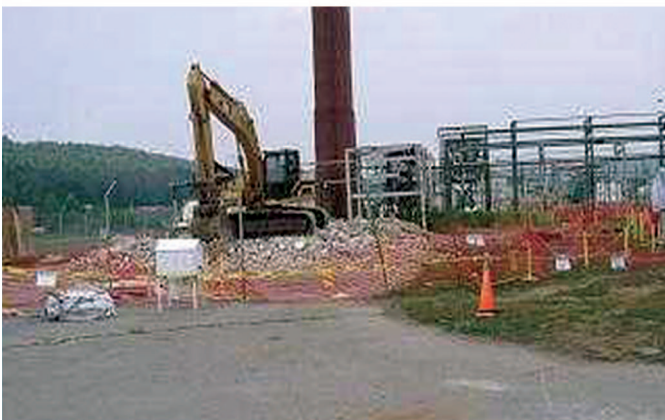
During D&D. Facility demolition nearing completion.
