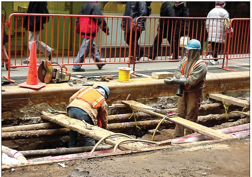
Figure 19: Workers Conducting Street Repairs in Lower Manhattan
