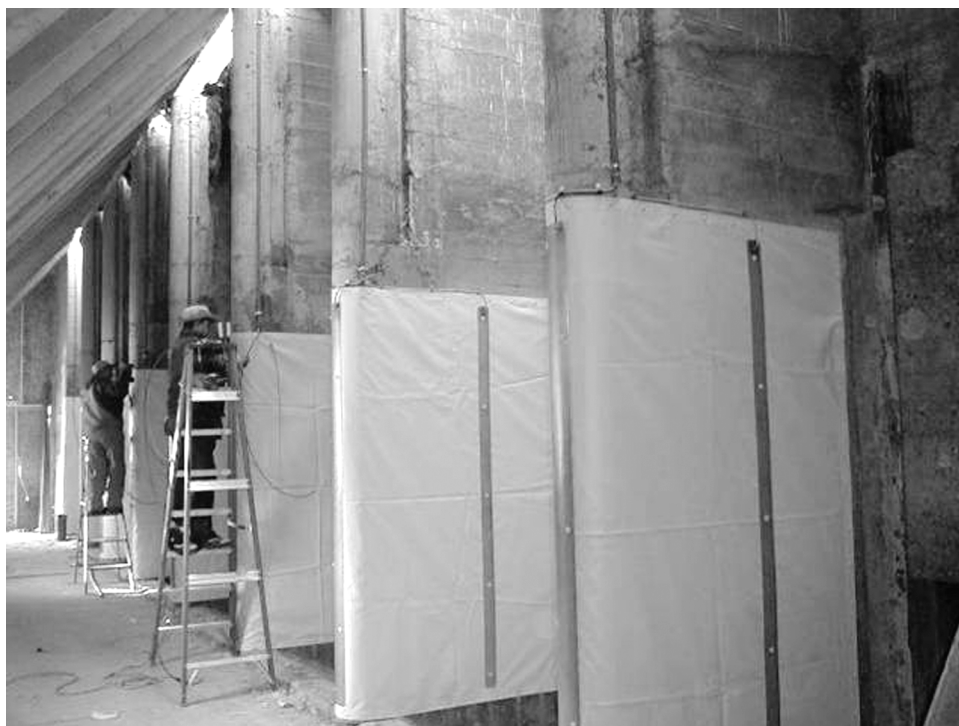
Figure 3: Workers Install Electric Fish Barrier Fabric on Canal Diversion Structure
