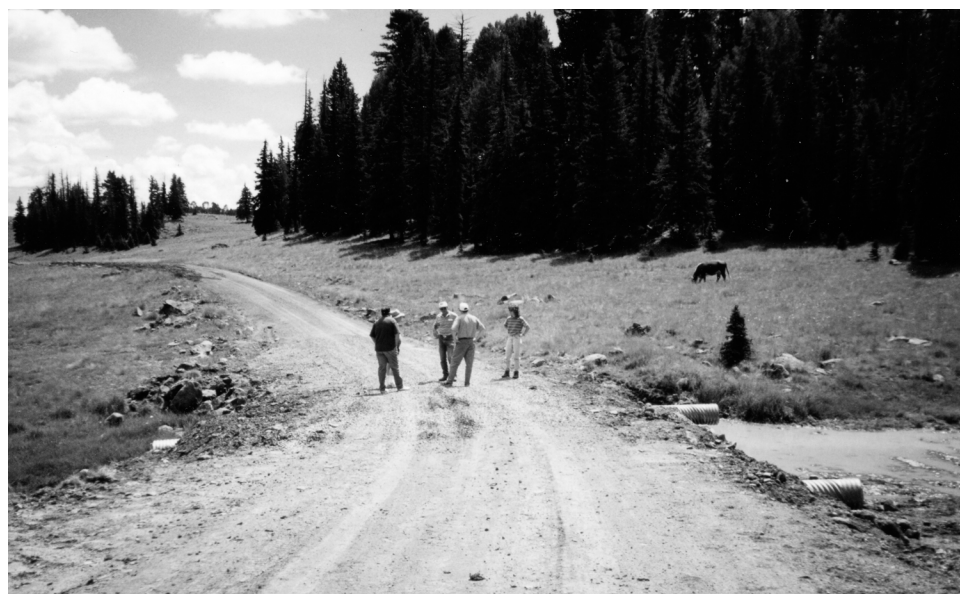
Figure 7: Site Visit to Culvert Replacement Project on Forest Service Land
