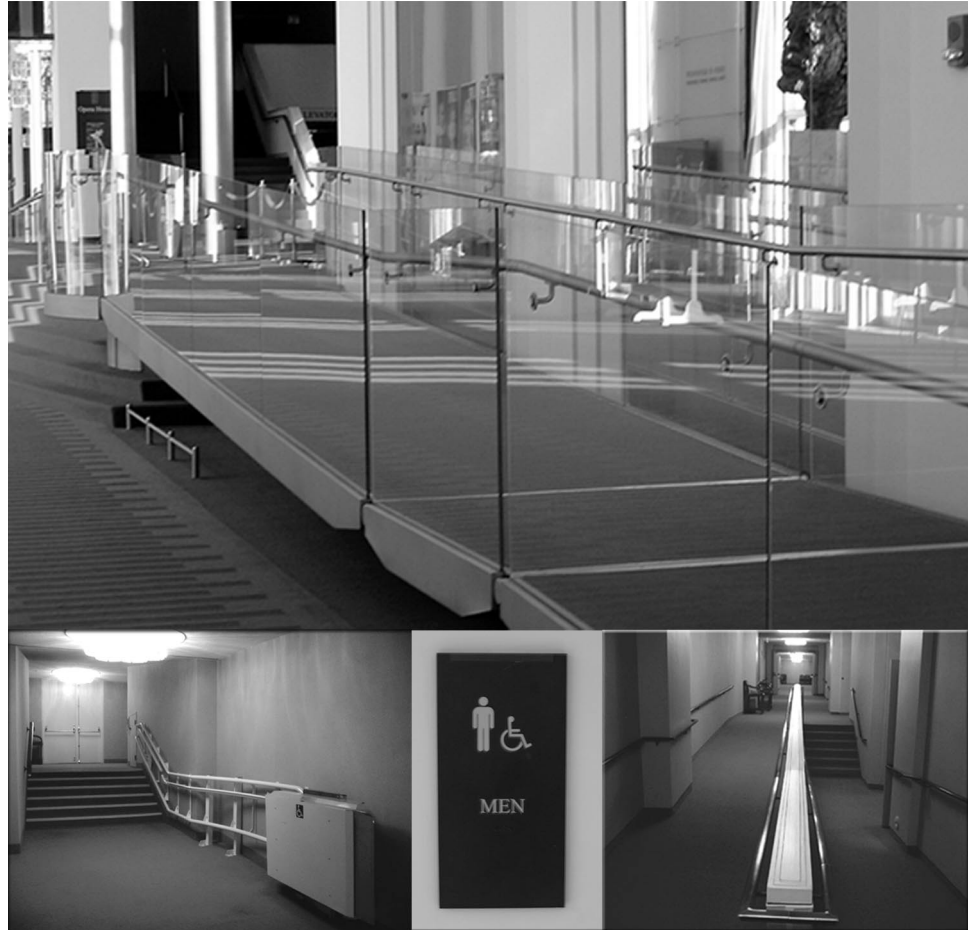
Figure 9: Selected Disabled Access Improvements to the Kennedy Center Made as Part of the Comprehensive Building Plan
