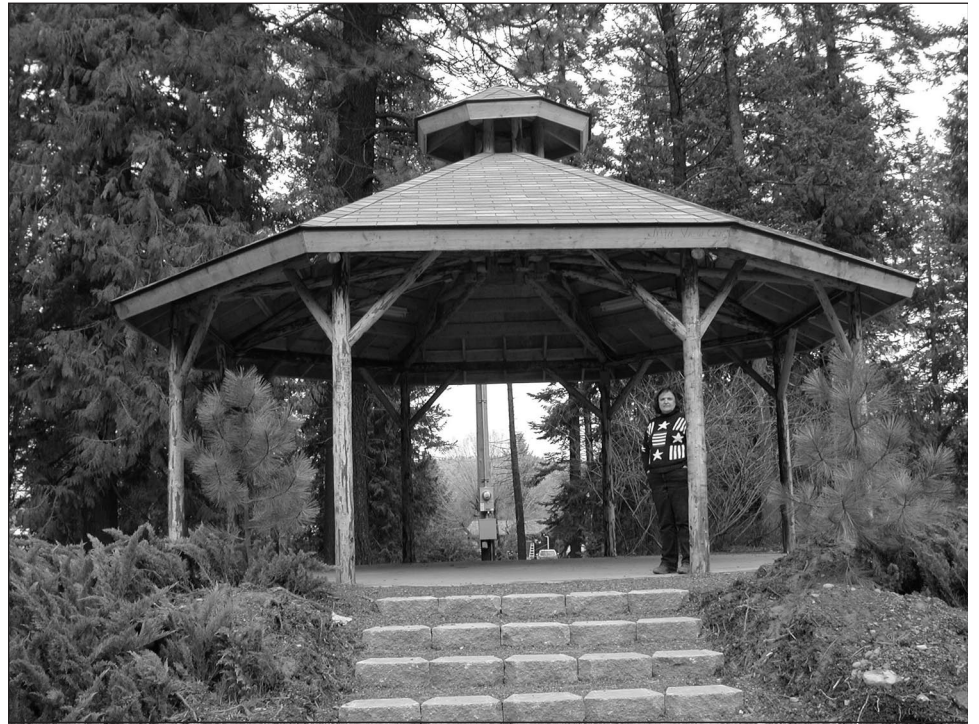
Figure 7: Kiosk Built from Roundwood and Small-Diameter Wood
