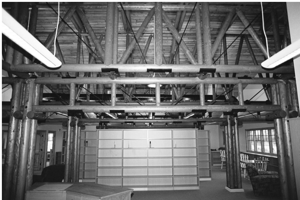
Figure 8: Interior of Darby Community Library Built from Roundwood, Darby, Montana
