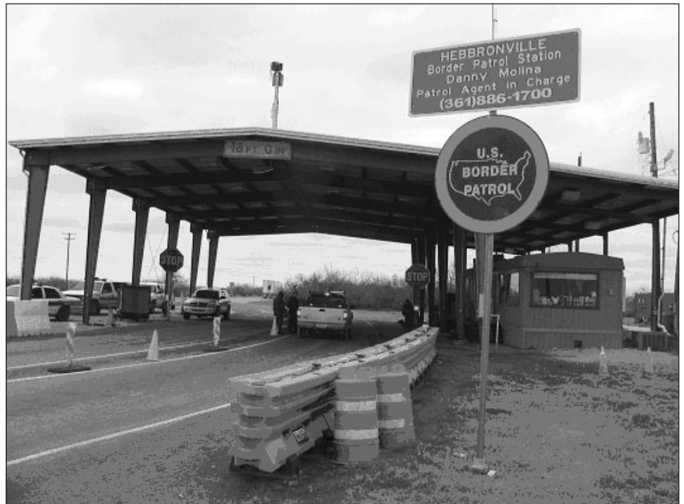
Figure 19: Permanent Checkpoint on State Highway 359 Near Hebronville, Texas
