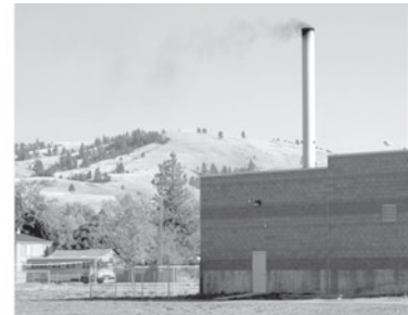
Wood-fired heating facility at rural school.
