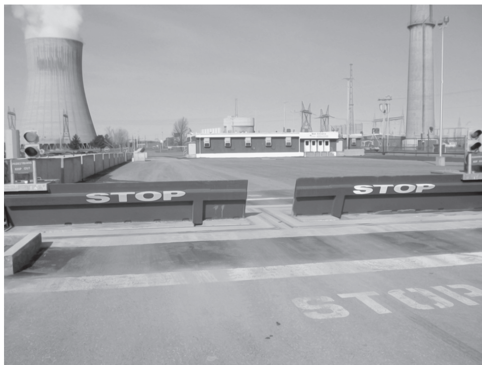
Figure 4: Example of an Active Vehicle Barrier System
