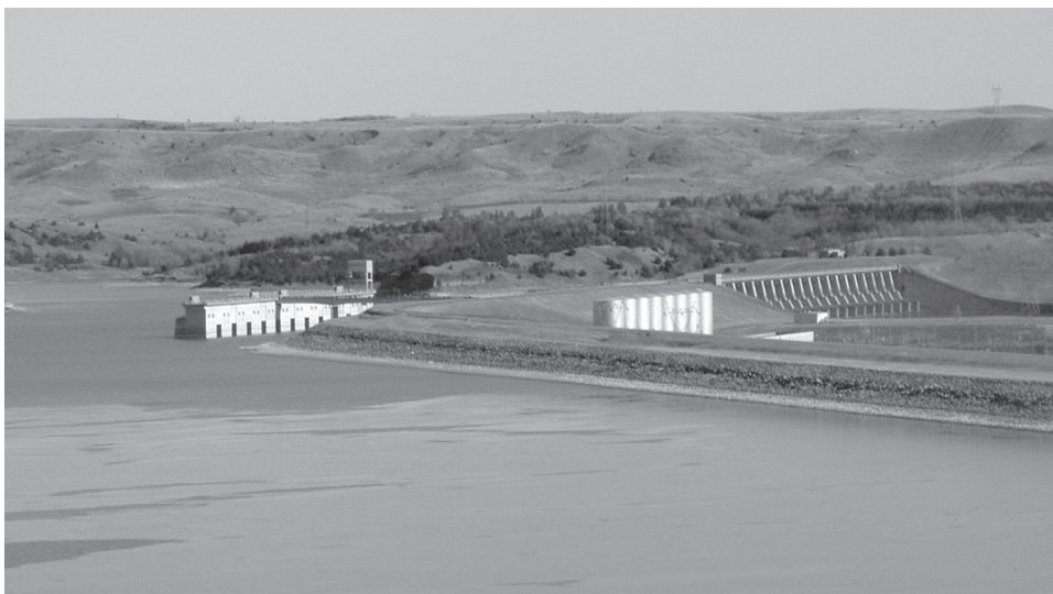
Figure 1: The Fort Randall Dam and Lake Case (February 2006)
