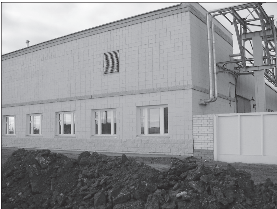
Figure 2: Completed Firehouse at Shchuch'ye, November 2005
