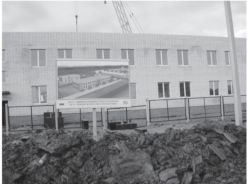
Figure 3: Administration/Cafeteria Building under Construction, November 2005
